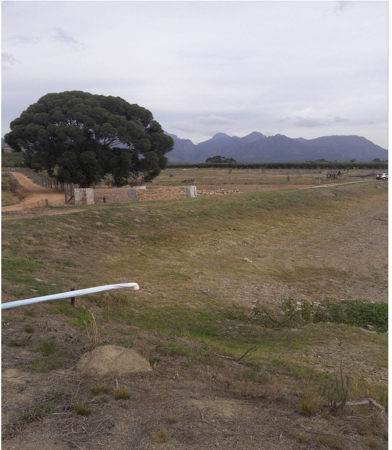
Photo 3: View on entrance from dam wall and entrance gate
