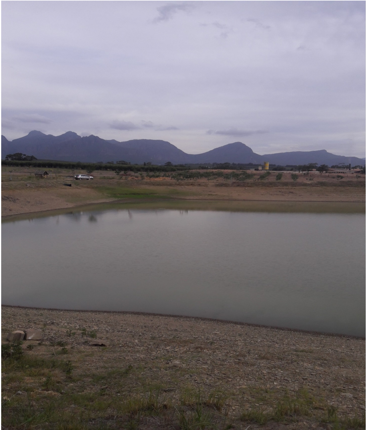
Photo 4: View across from dam wall where Conference building is to be built Brickfields in background
