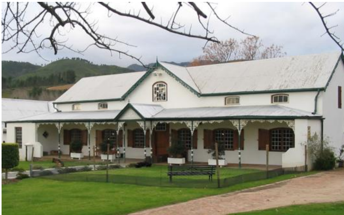
Figure 11: Victorianized Dutch Colonial homestead: Nabygelegen, Bovlei, Wellington. The earlier central and side gables were clipped and a corrugated iron roof and verandah added. (Photo: Graham Jacobs: August 2005).
