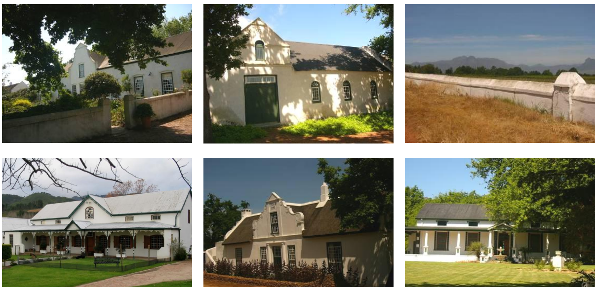
Figure 22a: Representative images of the Lower Berg River Valley illustrating a farm werf architecture which is typically more formal, ordered and decorative by comparison with the rural architecture of the Upper Berg River Valley in terms of the layout of farm building, the use of low walls to enclose the werf space, the presence of front and end gables, the use of later decorative veranda elements, and a pattern of oak tree planting around the werf.
