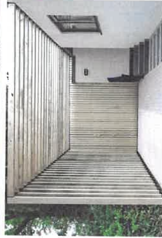
Figure 48: Timber and steel structure carports.
