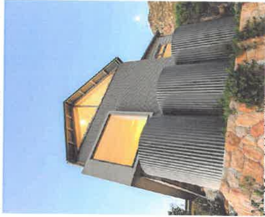
Figure 46: Timber slats used to conceal rainwater harvesting tanks
