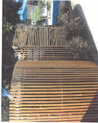
Figure 46: Timber slats used to conceal rainwater harvesting tanks
