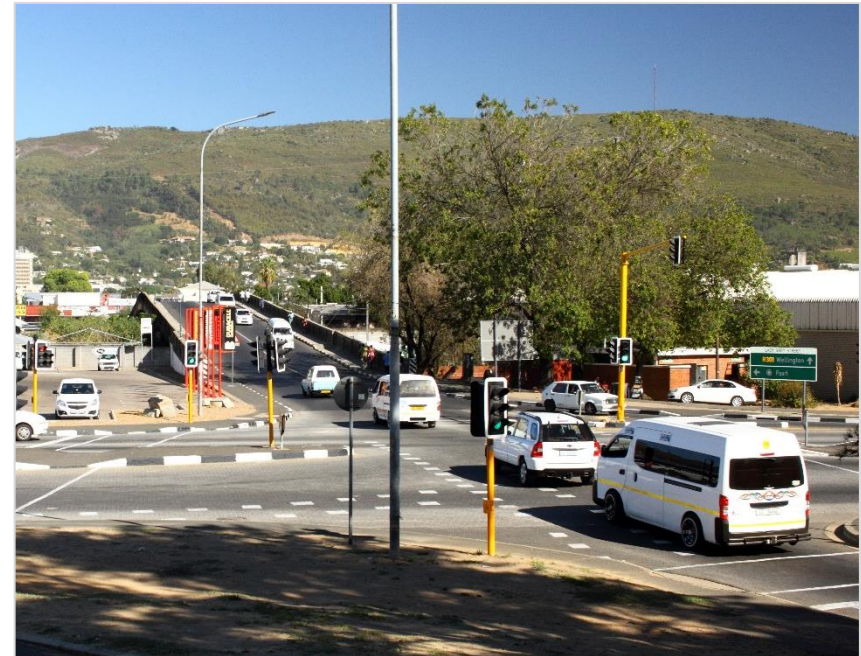
Photograph 2: Lady Grey Street Road Over Bridge
