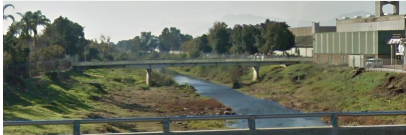
Figure 24: Existing Pedestrian Bridge Between Huguenot Station and Old Rembrandt Mall
