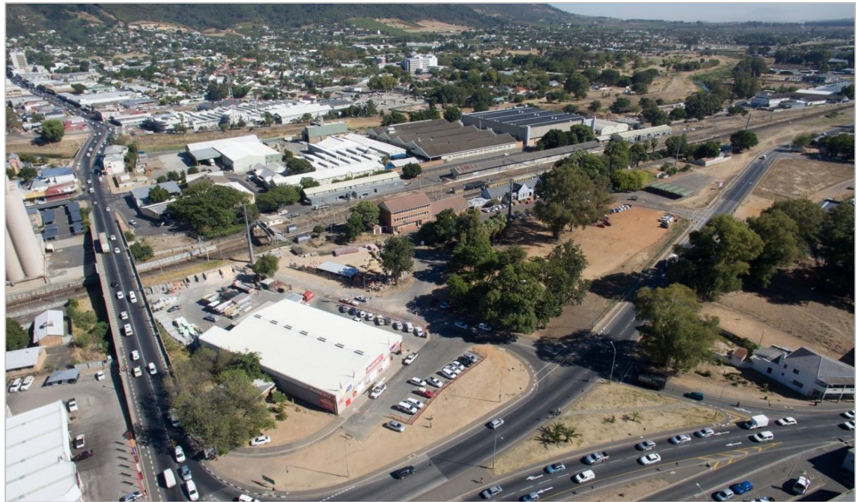
Photograph 7: Huguenot Station Precinct
