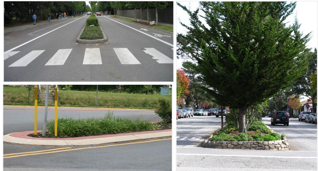
Figure 43: Landscaped Medians Contributing towards the Surrounding Character
