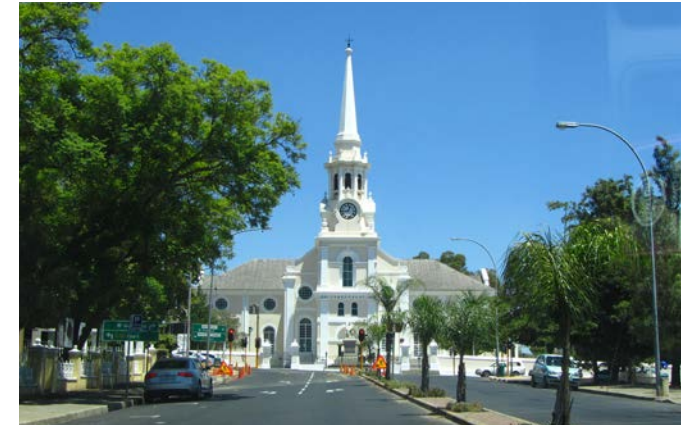
PHOTO 9. THE NG CHURCH ON THE AXIS OF CHURCH STREET, WELLINGTON IS AN IMPORTANT LANDMARK FEATURE
