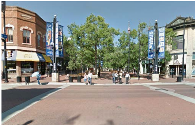
PHOTO 51. RAISED AND PAVED LEVEL PEDESTRIAN CROSSING - PEARL STREET, BOULDER, COLORADO
