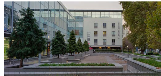
PHOTO 42. LANDSCAPED FORECOURT SPACE- CLAREMONT LIBRARY (DHK ARCHITECTS)
