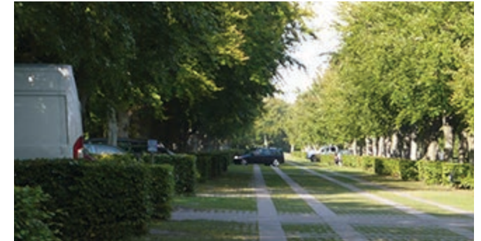
PHOTO 53. TREADED, MULTI-FUNCTIONAL PARKING COURT
