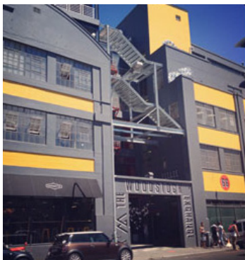
PHOTO 34. LANDMARK RENOVATED WAREHOUSE
