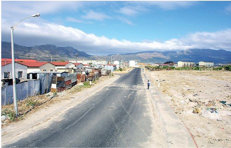
Level 3 Unacceptable standard of cleanliness
