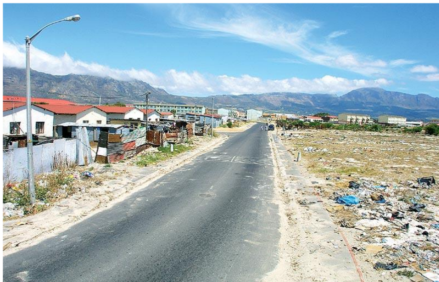
Level 4 Totally unacceptable standard of cleanliness
